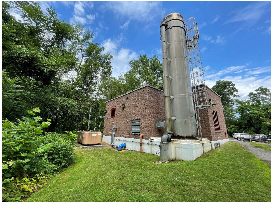
Photo 4. Well 4 & 4A Enclosure
