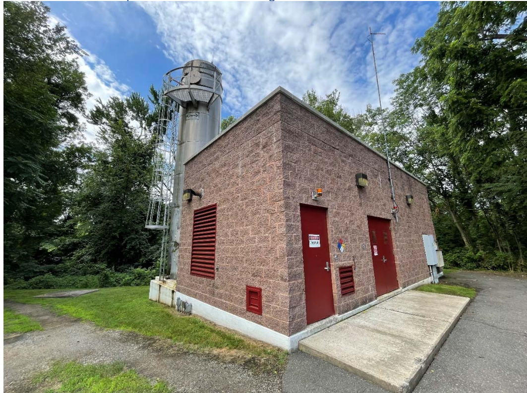
Photo 3. Well 4 & 4A Enclosure
